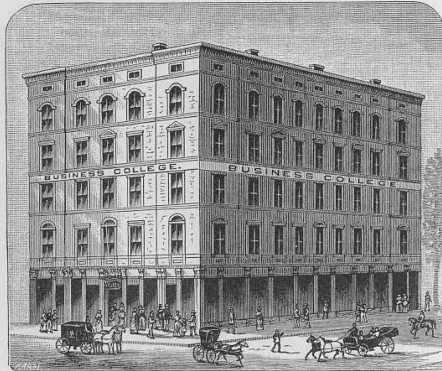
The College Building in New York City, where Mr. Spencer's last Course of Instruction was given, in 1864.
